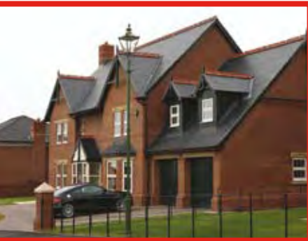
Wensley Roofing has roofed many houses at the prestigious Wynyard site near Stockton.
