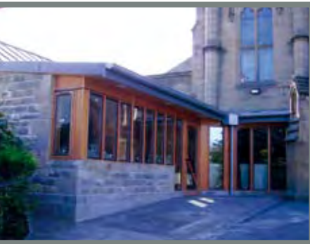
New entrance, office and toilets at St Mary's Catholic Church, Hexham.
