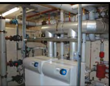
Supply and installation of new boilers.
