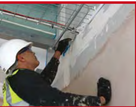
Isoler provides the highest possible quality of workmanship.
