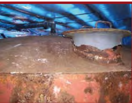
Contaminated vessel at Newcastle brewery after asbestos removal but prior to cleaning.
