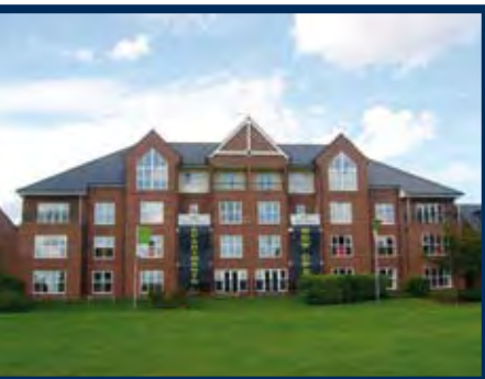
Luxury apartment block in Durham with natural slate roofing.
