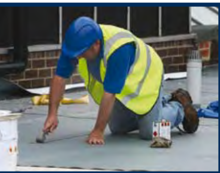
Applying single-ply membrane - one of the comprehensive range of services supplied by Springs Roofing.
