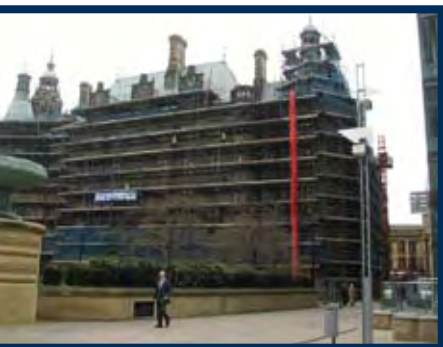
Sheffield Town Hall - complete reroofing including leadwork, copper dome and lightning protection.
