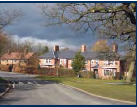
Jennings Roofing is contracted by the Ministry of Defence to work at Catterick, the UK's biggest army base.
