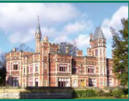
Saltwell Towers, Gateshead - structural stabilisation of historic Grade 1 listed building.
