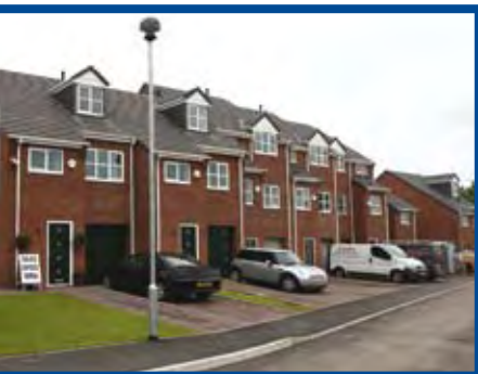
Roof Truss supplied the trussed rafters for this new housing development at Chester-le-Street.
