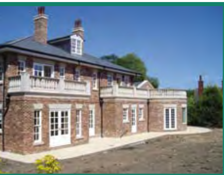
Potters Bank, Durham - new build of six bedroom dwelling with swimming pool, spa, gym and cinema.
