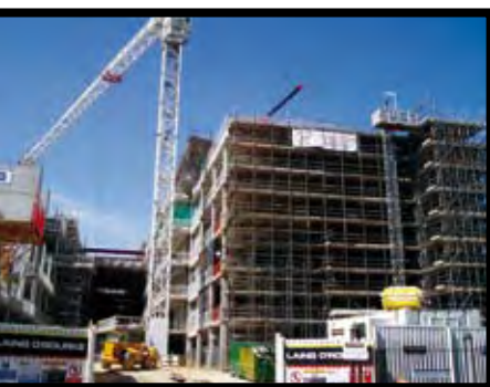
Installation of a specialist cast iron drainage system at the Royal Victoria Infirmary in Newcastle.
